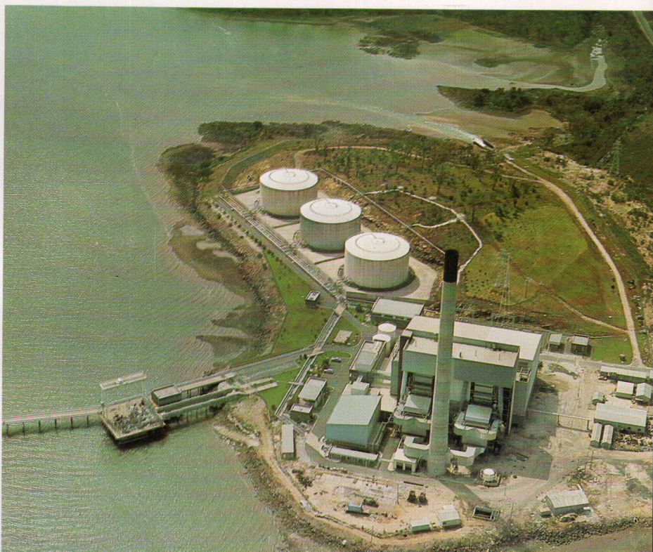
Tasmania's only thermal electricity generating station at Bell Bay
