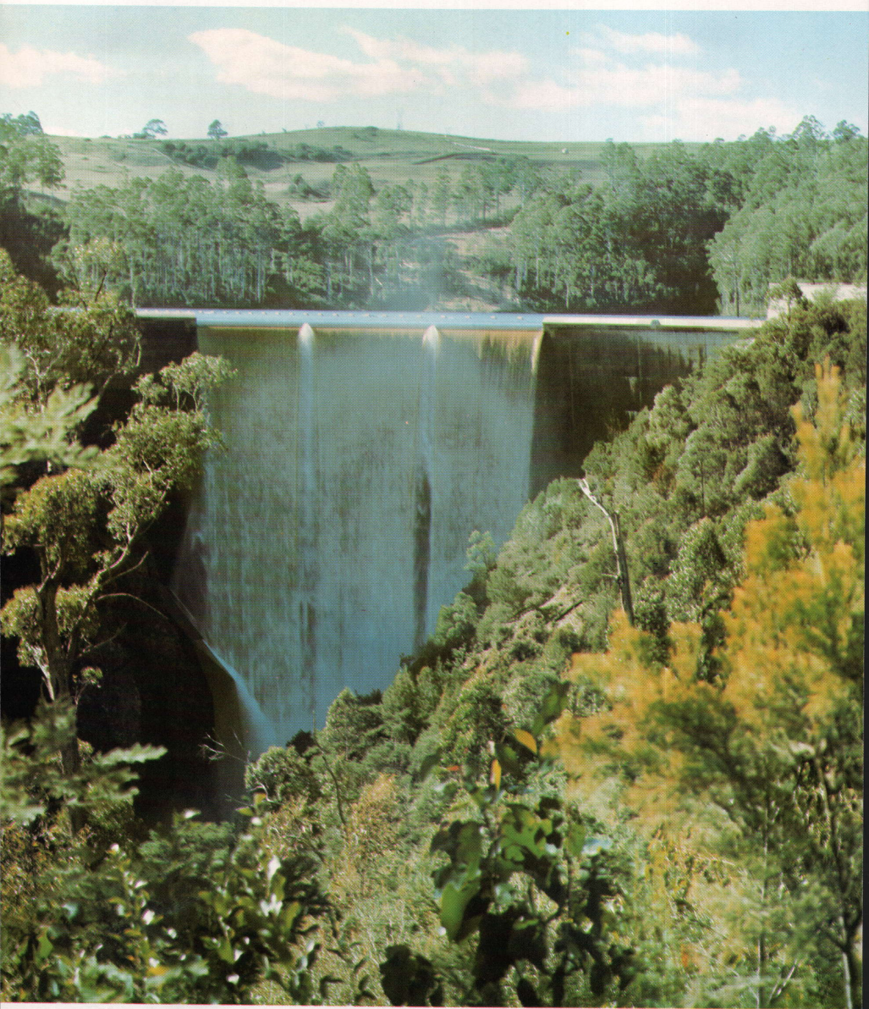
Devil's Gate Dam (84 metres) holding back the waters of Lake Barrington on the River Forth
